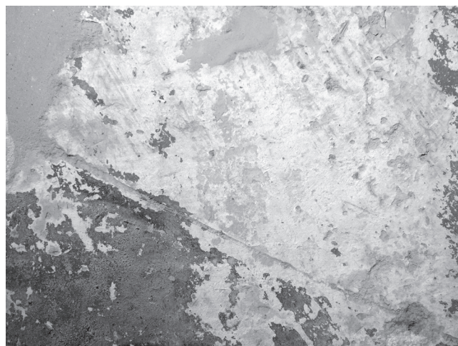
Fig. 6 Detail of a wall painting with missing paint layer, the white ground has become visible, source: Alexandra Skedzuhn 2011
