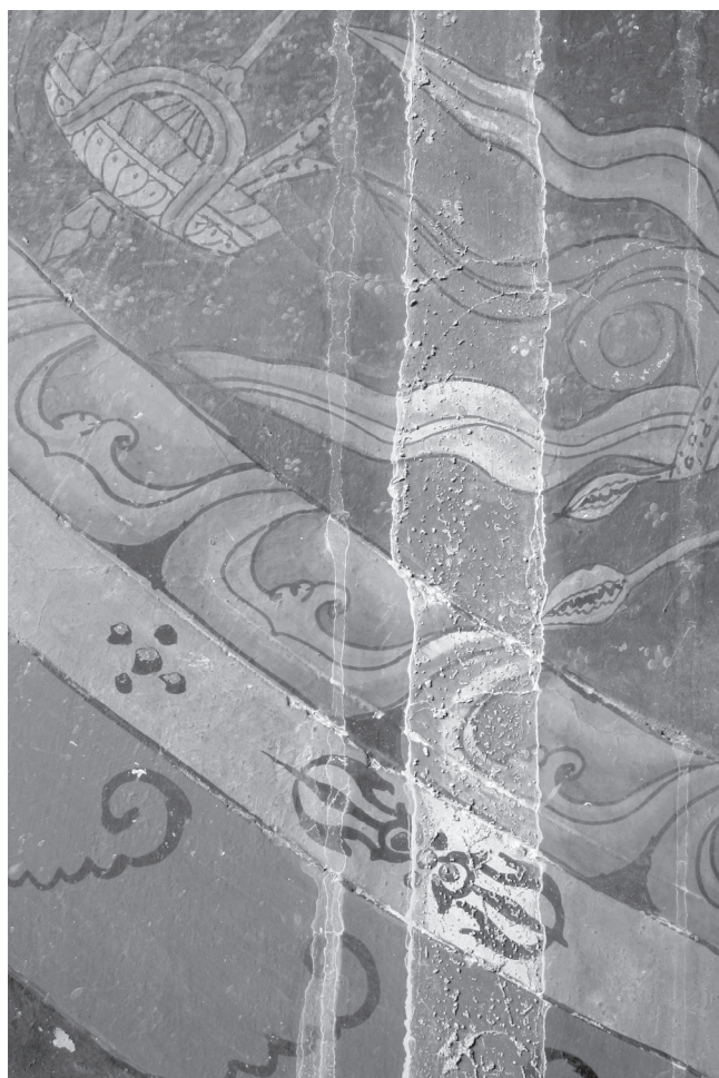
Fig. 16 Orpiment underpainting visible due to water infiltration which has washed away the overlying ochre, source: Steven Post 2006
